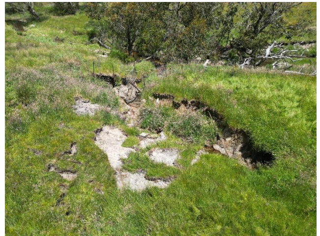
Figure 3 Before the works
