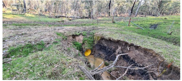
Figure 2. Post fire, the deepening of the creek meant that access to the half the property was cut off. Previous crossing attempts had multiple failures and caused large amounts of sediment to move down stream
